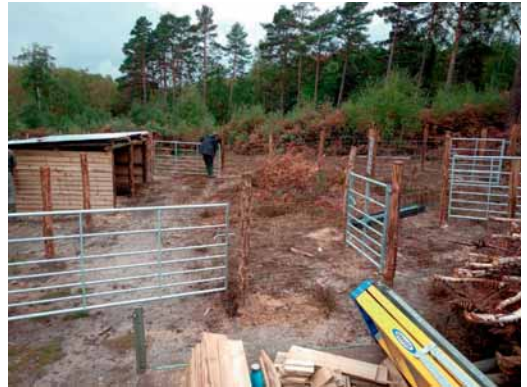
A view of the completed enclosure
