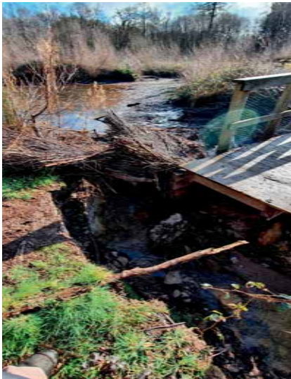
Photos A and B show the large leak in the pond adjacent to the bridge. The wood bundles we have been using to stem the flow can be seen, however the drop in water level (Photo C) is dramatic and a long-term solution is urgently needed.
