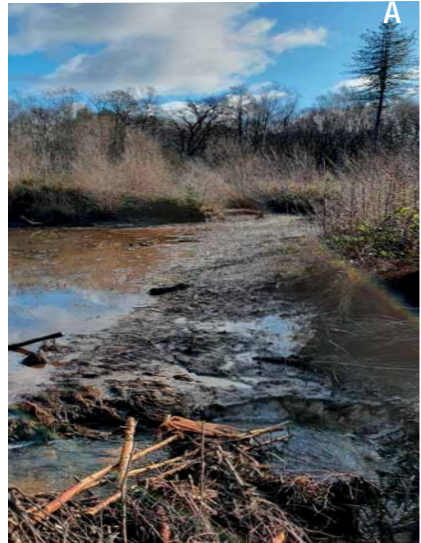
Photos A and B show the large leak in the pond adjacent to the bridge. The wood bundles we have been using to stem the flow can be seen, however the drop in water level (Photo C) is dramatic and a long-term solution is urgently needed.
