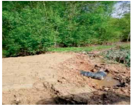
An outflow pipe has been installed to ensure excess water can run out of the pond in a controlled way.
