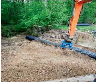
An outflow pipe has been installed to ensure excess water can run out of the pond in a controlled way.
